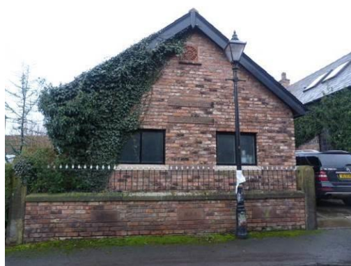
Boundary treatment and gate posts characteristic of the wider area in front of the former Chapel
