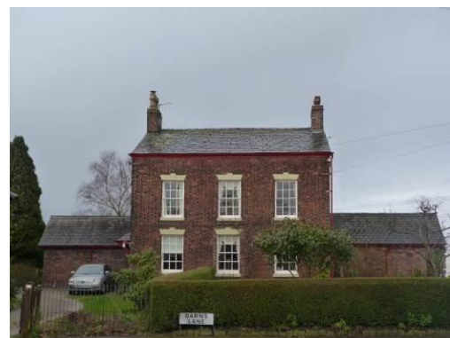
1-2 Greenbank, which was originally one large dwelling but has subsequently been divided into two
