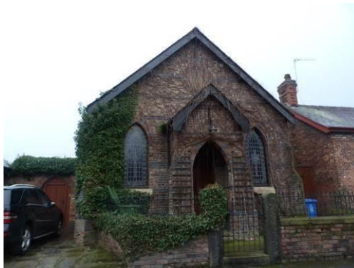
Former Methodist Chapel, which has been converted into a residential dwelling
